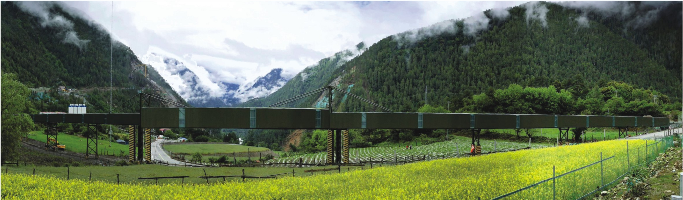
The fully enclosed off-road belt conveyor passes through the nature reserve in a safe and environmentally friendly manner.
