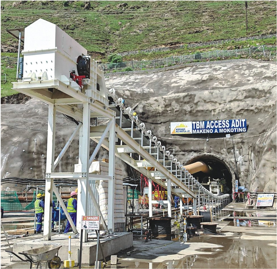
The 35km ultra-long-distance continuous belt conveyors boost the construction of the Lesotho Highlands Water Project.
