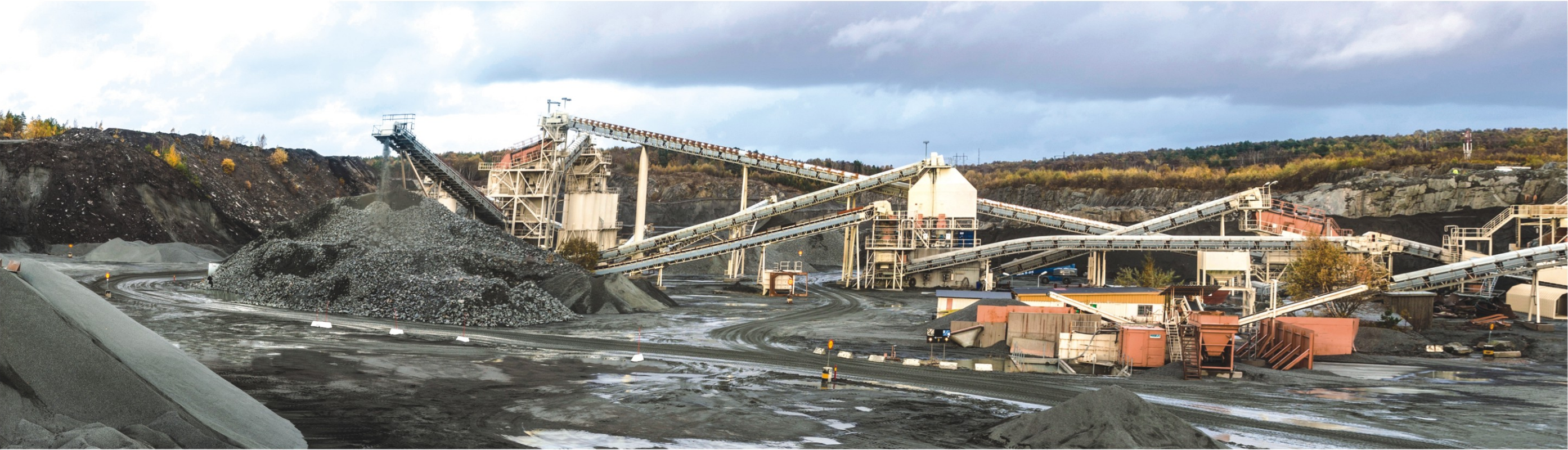
Small gravel yards realize the local utilization of crushed stone resources.
