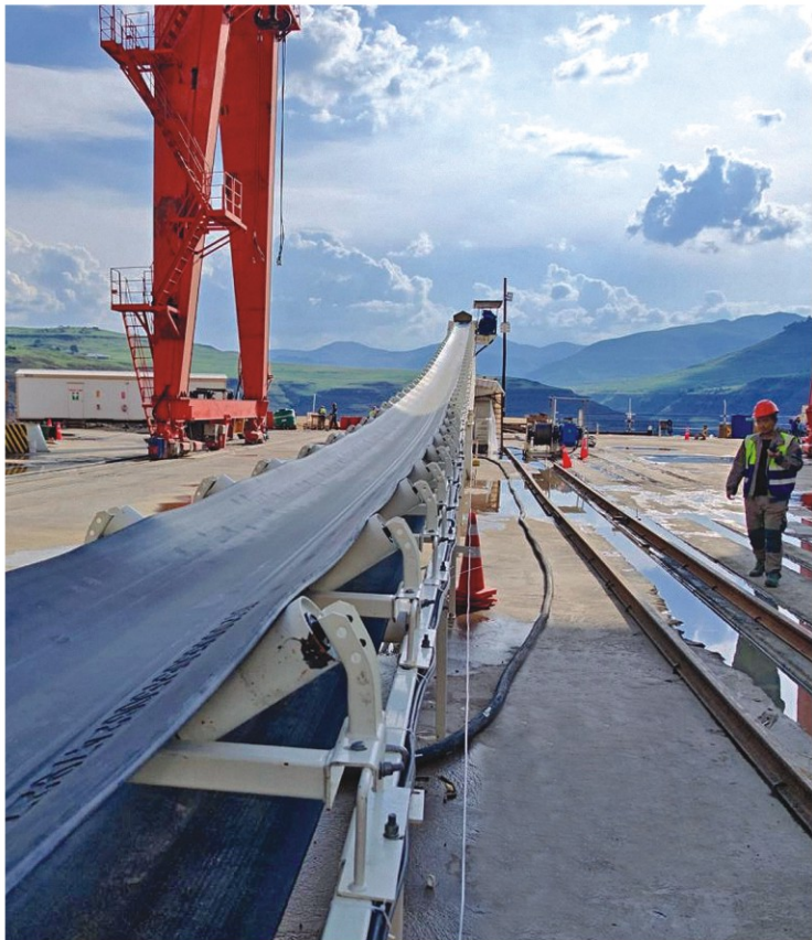
The 35km ultra-long-distance continuous belt conveyors boost the construction of the Lesotho Highlands Water Project.
