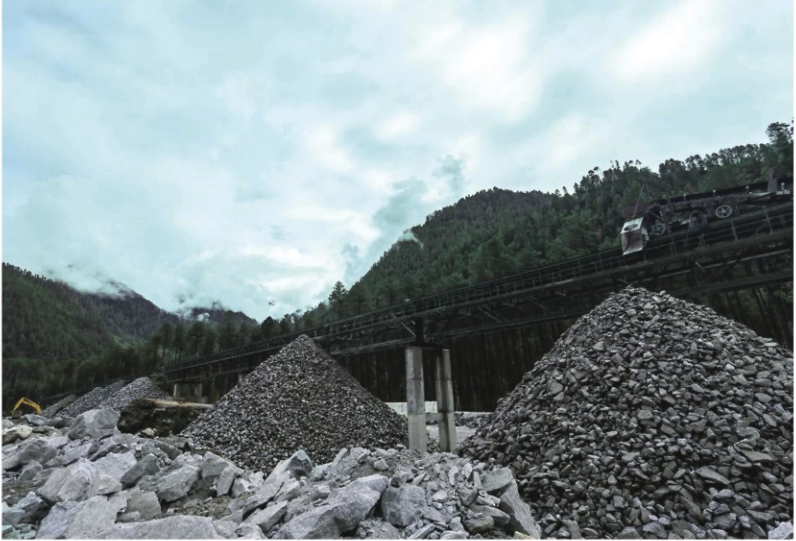
The tripper car achieves continuous material distribution.
