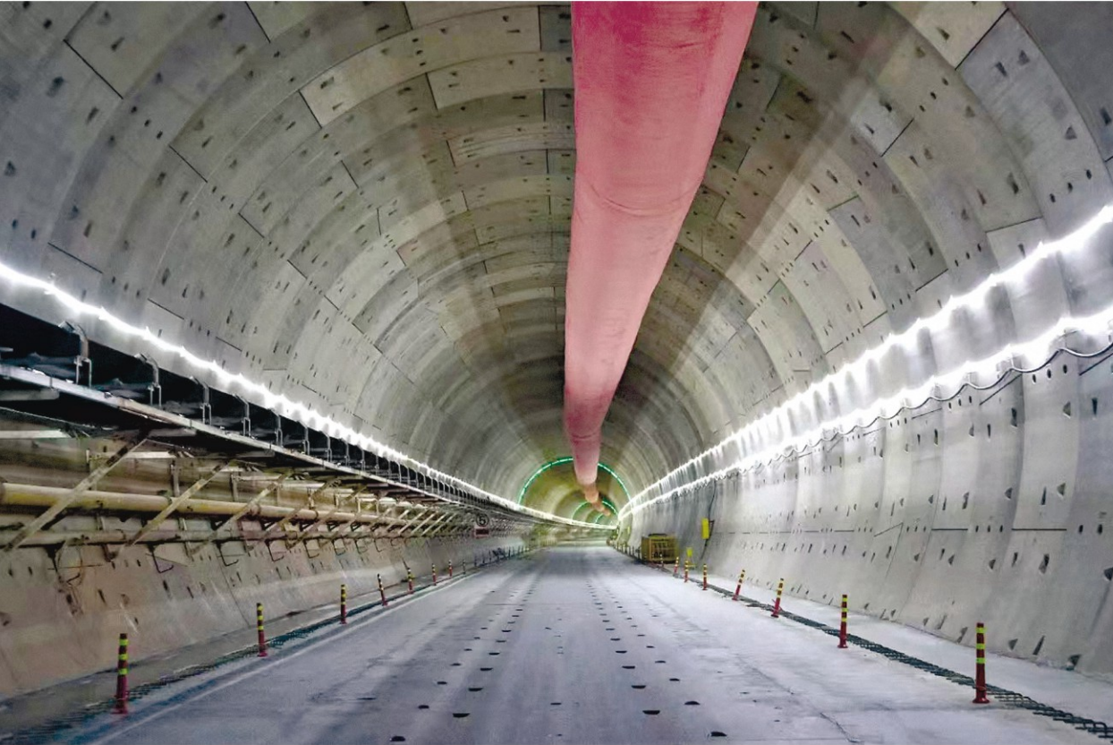
Long-distance continuous belt conveyor boosts the construction of Zhuhai-Zhaoqing High-speed Railway Project.
