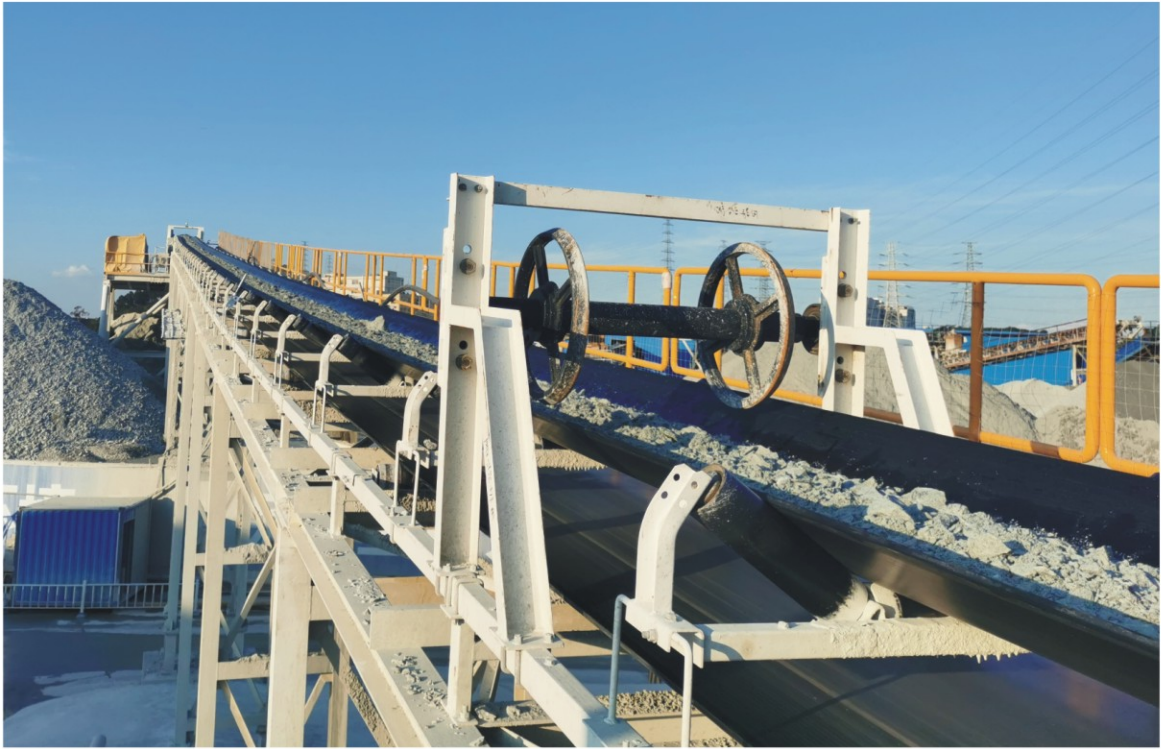
Ultra-long continuous belt conveyor boosts the construction of the Pearl River Delta Water Resources Allocation Project.
