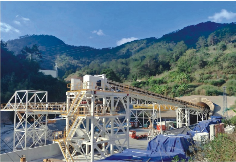
Ultra-long continuous belt conveyor boosts the construction of the Yangtze River Diversion Project.
