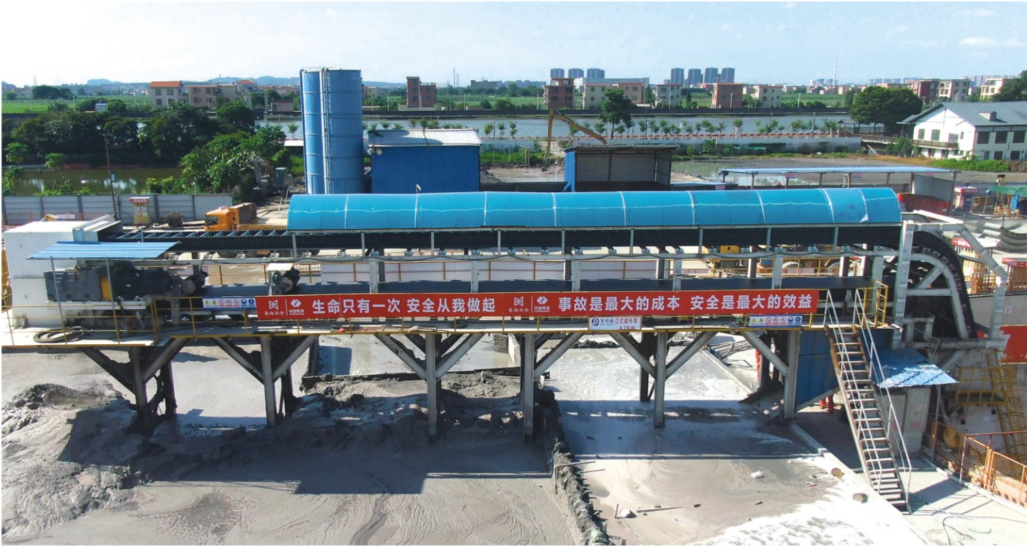
First-time achievement of continuous vertical transportation in a 75m ultra-deep shaft.
