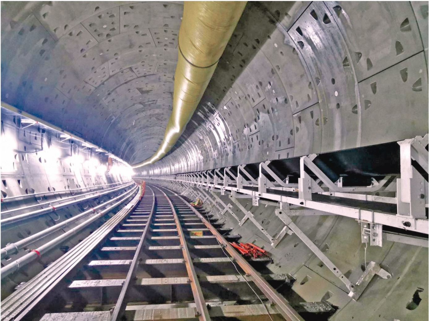
Adjustable idler frames are used for small-turn curves.
