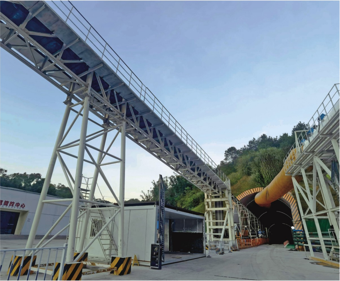
Ultra-long continuous belt conveyor boosts the construction of the Yangtze River Diversion Project.
