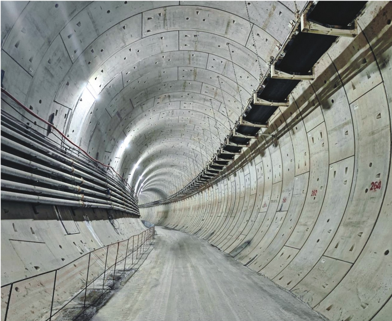
90°turning of multiple curves by a single conveyor is realized.
