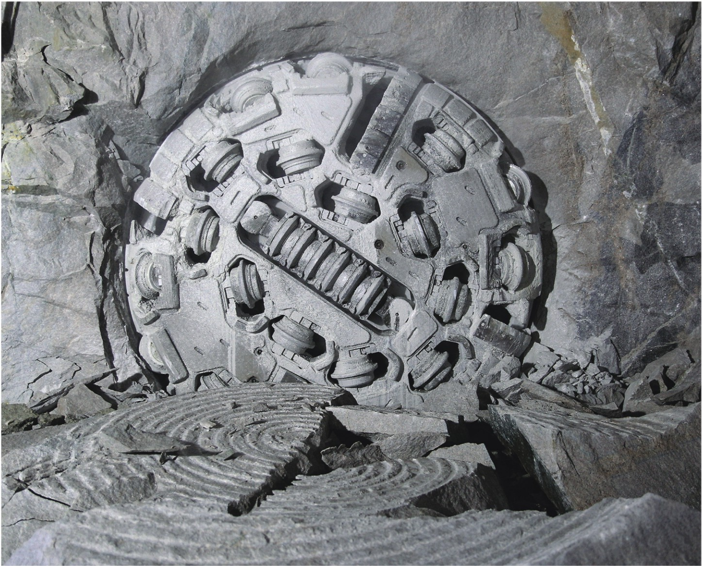
The TBM has achieved excellent performance in its debut.
