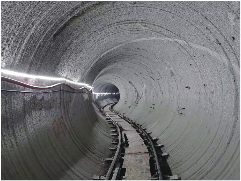
The TBM has negotiated several continuous small curves.
