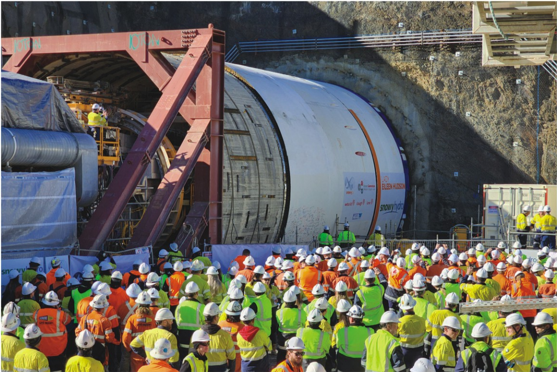
The launching of the TBM CREC-783 in Australia
