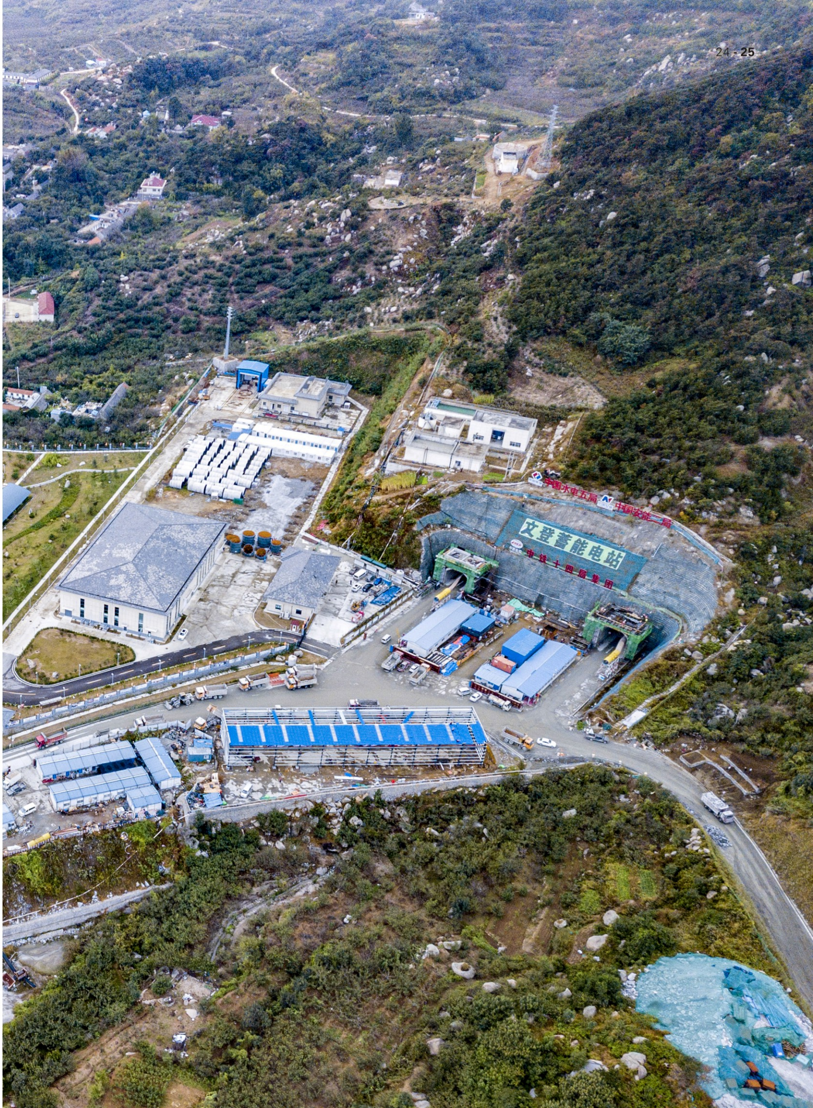
CREG has customized a compact TBM with a turning radius of 30 m for Wendeng Pumped Storage Power Station.
