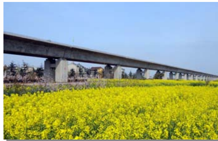
Beijing-Shanghai High Speed Railway
